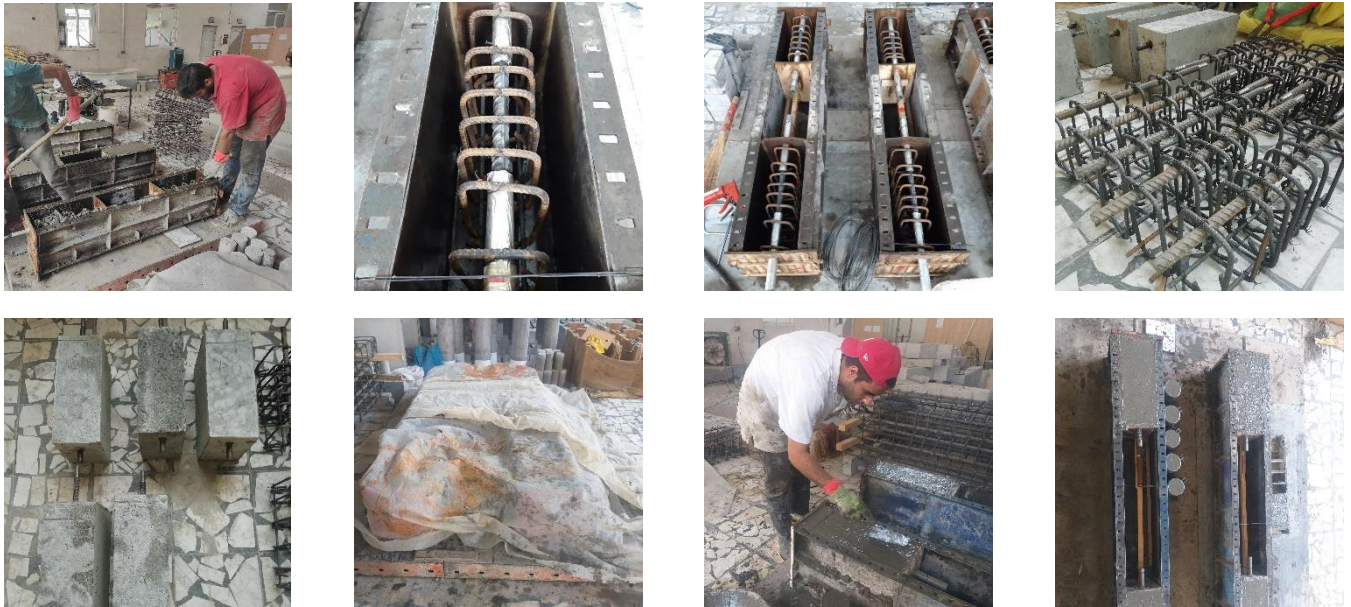
Fig. 4. Fabrication of reinforced concrete specimens
